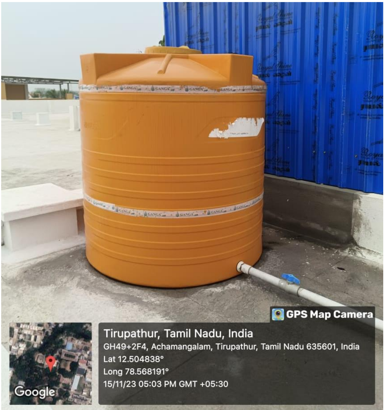
Roof top – MAW block
