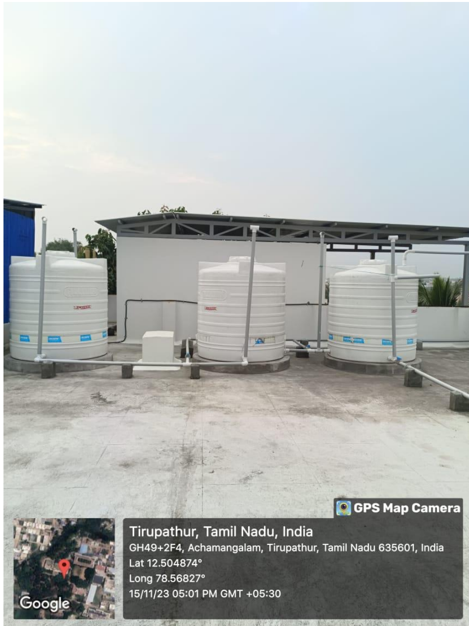
Roof top – MAW block
